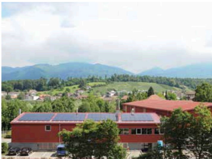
112 Panels à 290 Watt = 34,48kWp = 32'000kWh/Jahr
